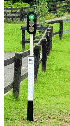
New mounting posts for The Signals
