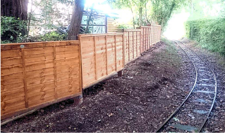
New fencing beside the Tram Track
