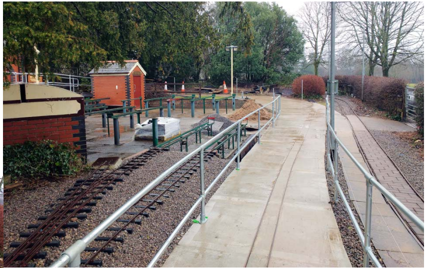
New approach path to the new bridge.
