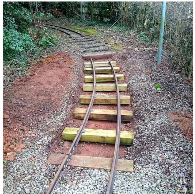
The tram track sleepers and rail replacement, part of an ongoing maintenance project
