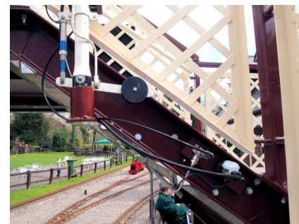
Members refitting the panels and adding the signalling furniture
