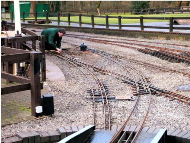
Work on the new point and crossover
