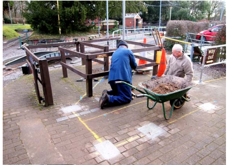
Tram maze footings being concreted
