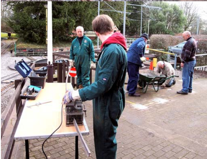
Rail bending to produce the correct curve radius
